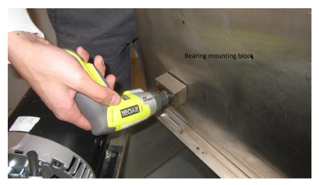
7. Pull the bearing mounting block off the roller shaft.
